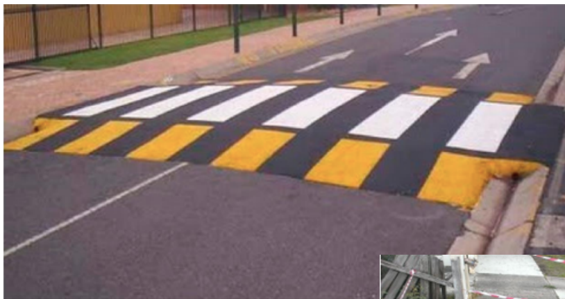
Fig 3.6 Raised humps on road for pedestrian crossing
