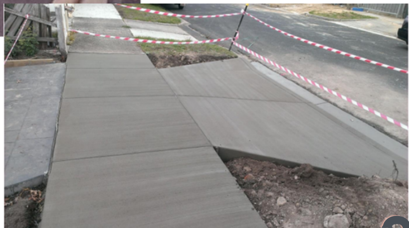
Fig 3.7 Homogeneous grit finish walkways
