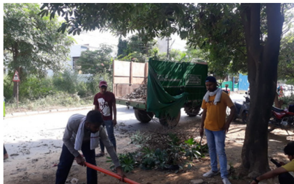
Cleaning and patch work
