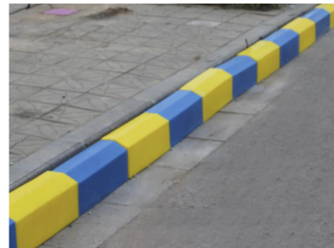
Fig 3.8 Walkways with kerb edging of accessible height
