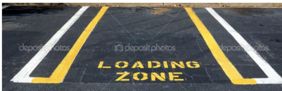
Fig 3.13 Lay By Lane Road Marking
