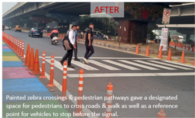
Painted zebra crossings & pedestrian pathways gave a designated space for pedestrians to cross roads & walk as well as a reference point for vehicles to stop before the signal.
